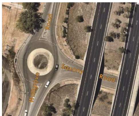
Figure 2: Intersection of Wallgrove Road with Saxony Road
